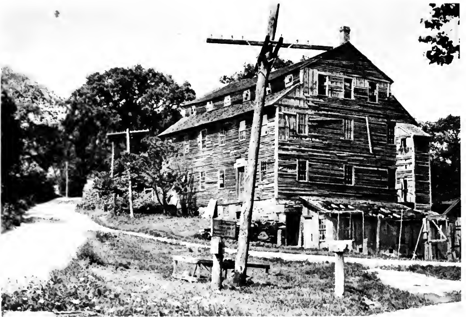
TWINE MILL, POMFRET LANDING
